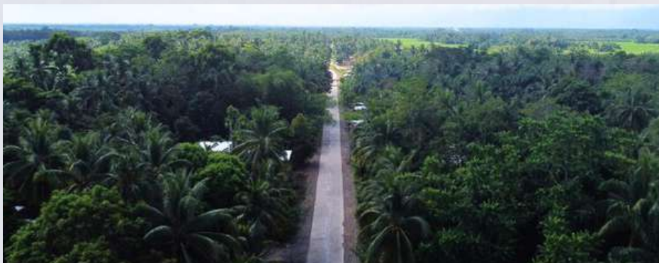
PDMU Conducts Simultaneous Final Project Inspection of FMR Project at Brgy. Salabaca, Esperanza, Sultan Kudarat on December 4, 2024
